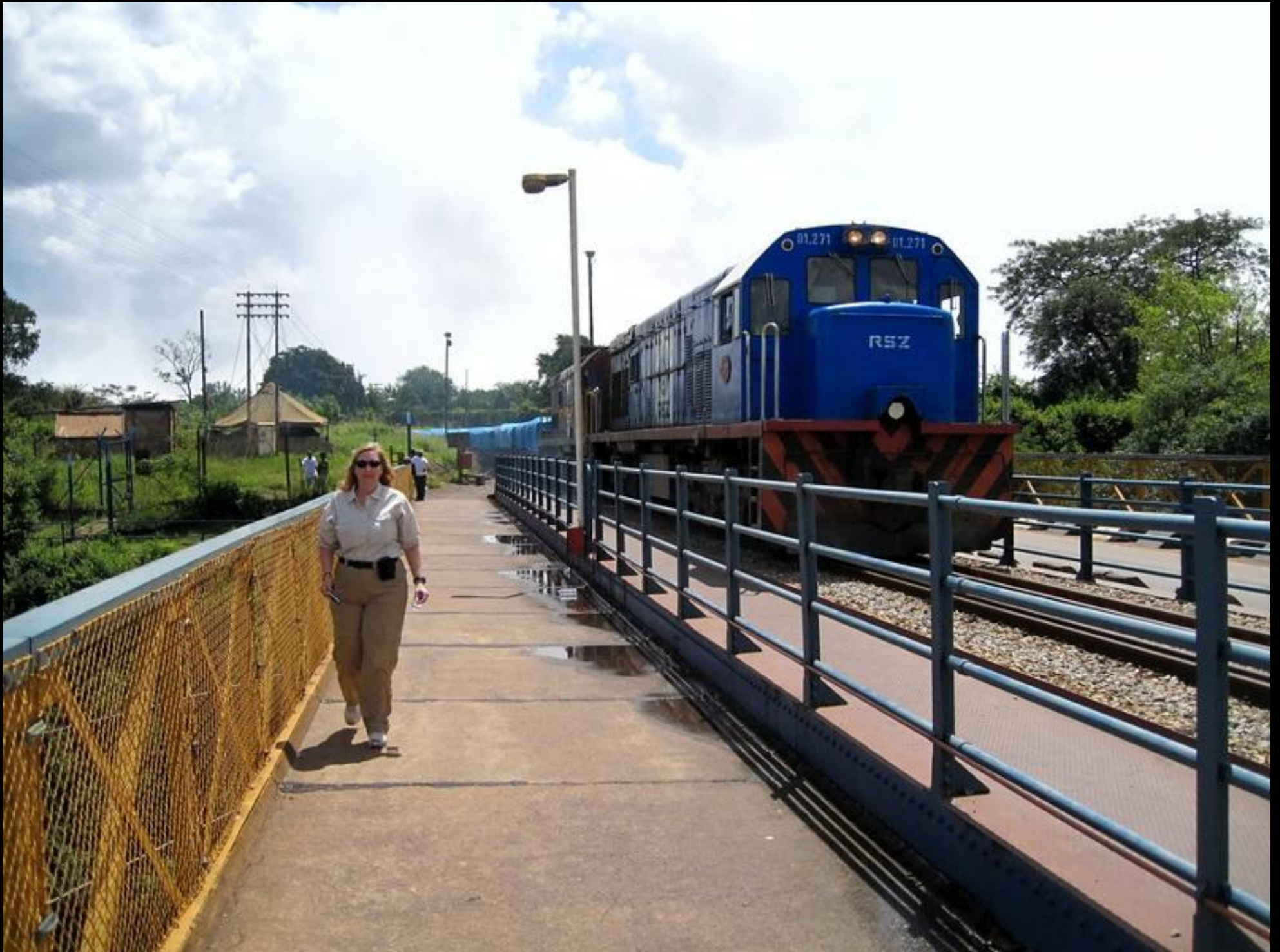
The Livingstone Bridge is rather old and shakes when the train crosses. There is room for a train, pedestrians and one lane of truck traffic. With this bridge Livingstone's dream of connecting Johannesburg to Cairo became true.
