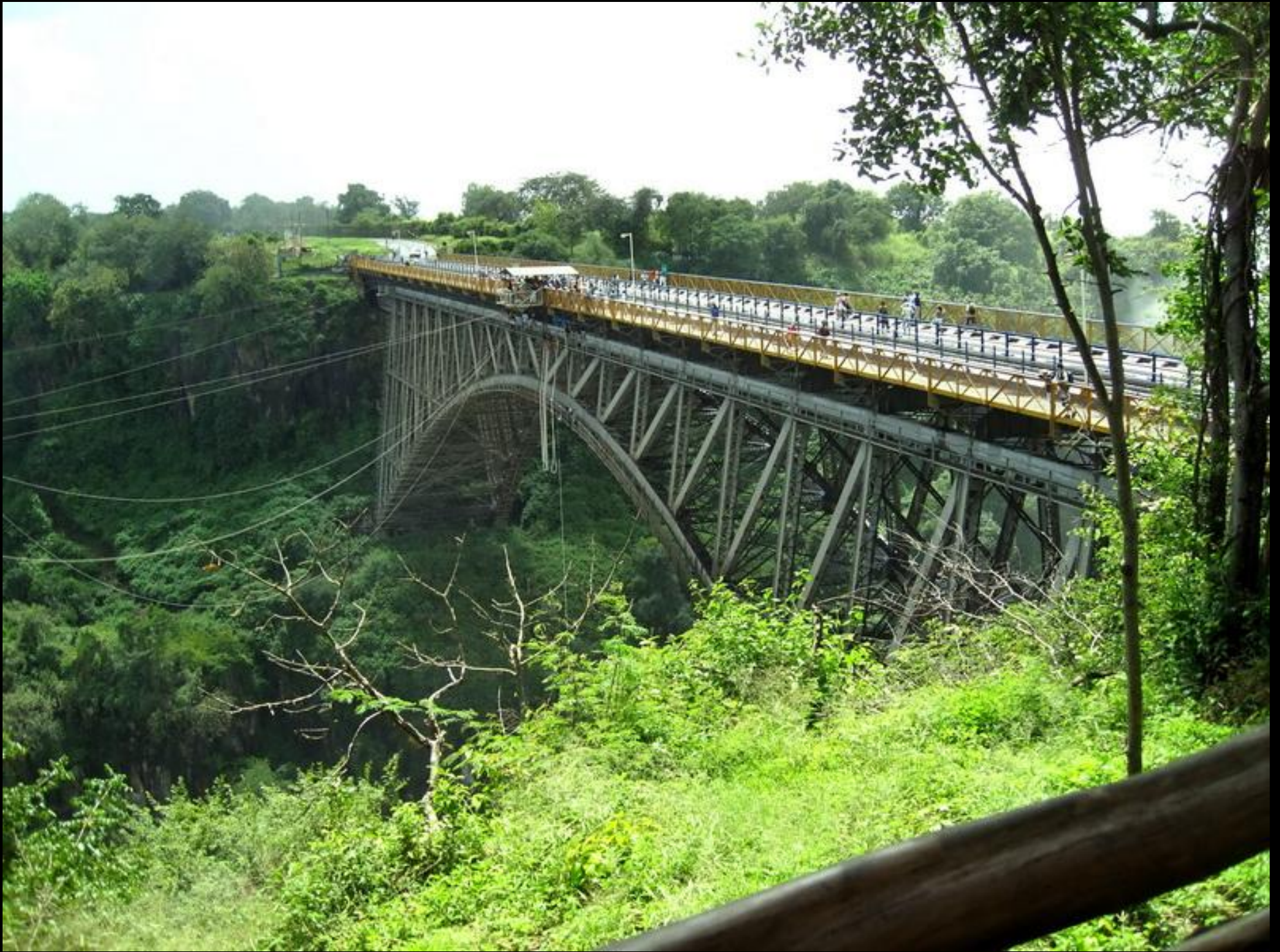
The platform in the middle of the bridge was the platform for the bungee jumpers. The cables were some of the different rides. One was a swing of sorts rather than a bungee jump.
