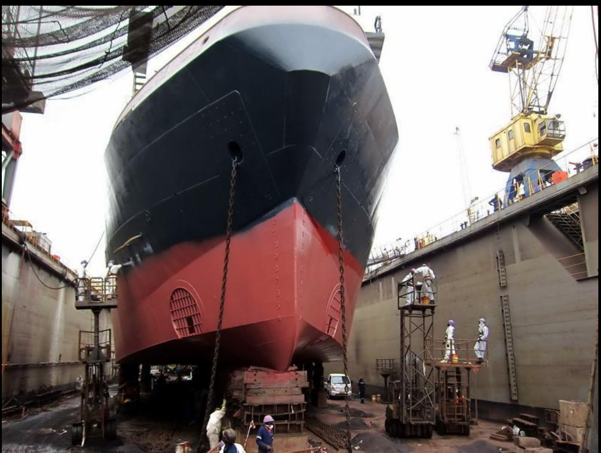
There is still one more coat of paint to go.
