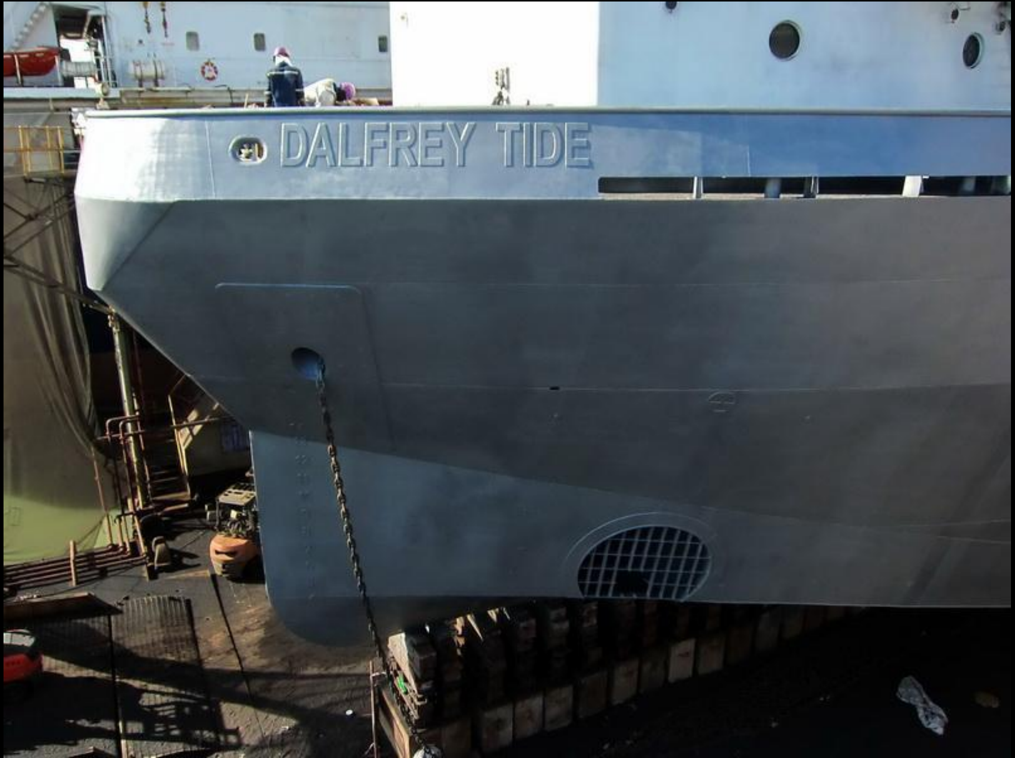
Primer coat complete, ready for painting
