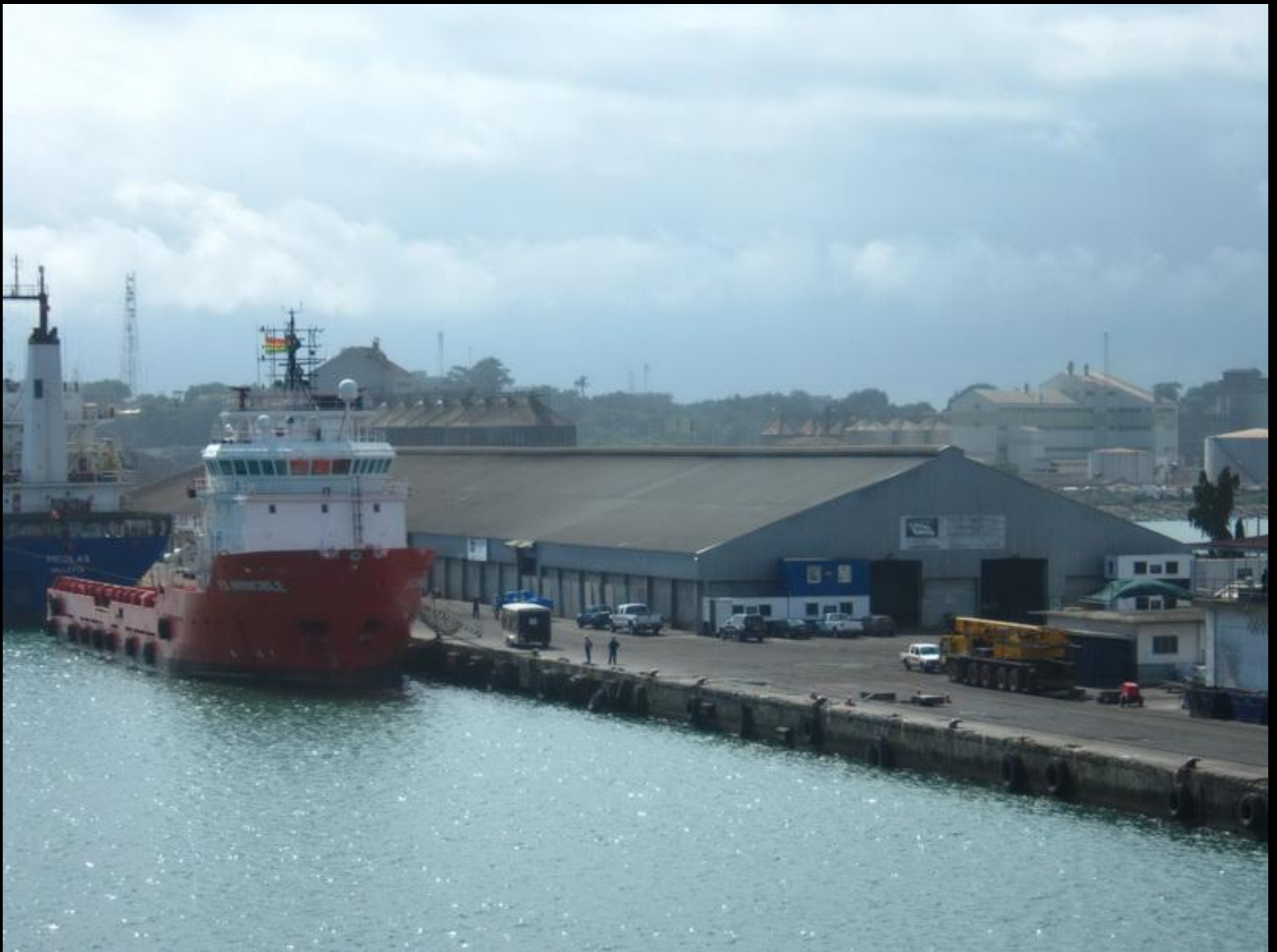
Here is one of four commercial warehouses in Takoradi containing ore and other products waiting to be exported.
