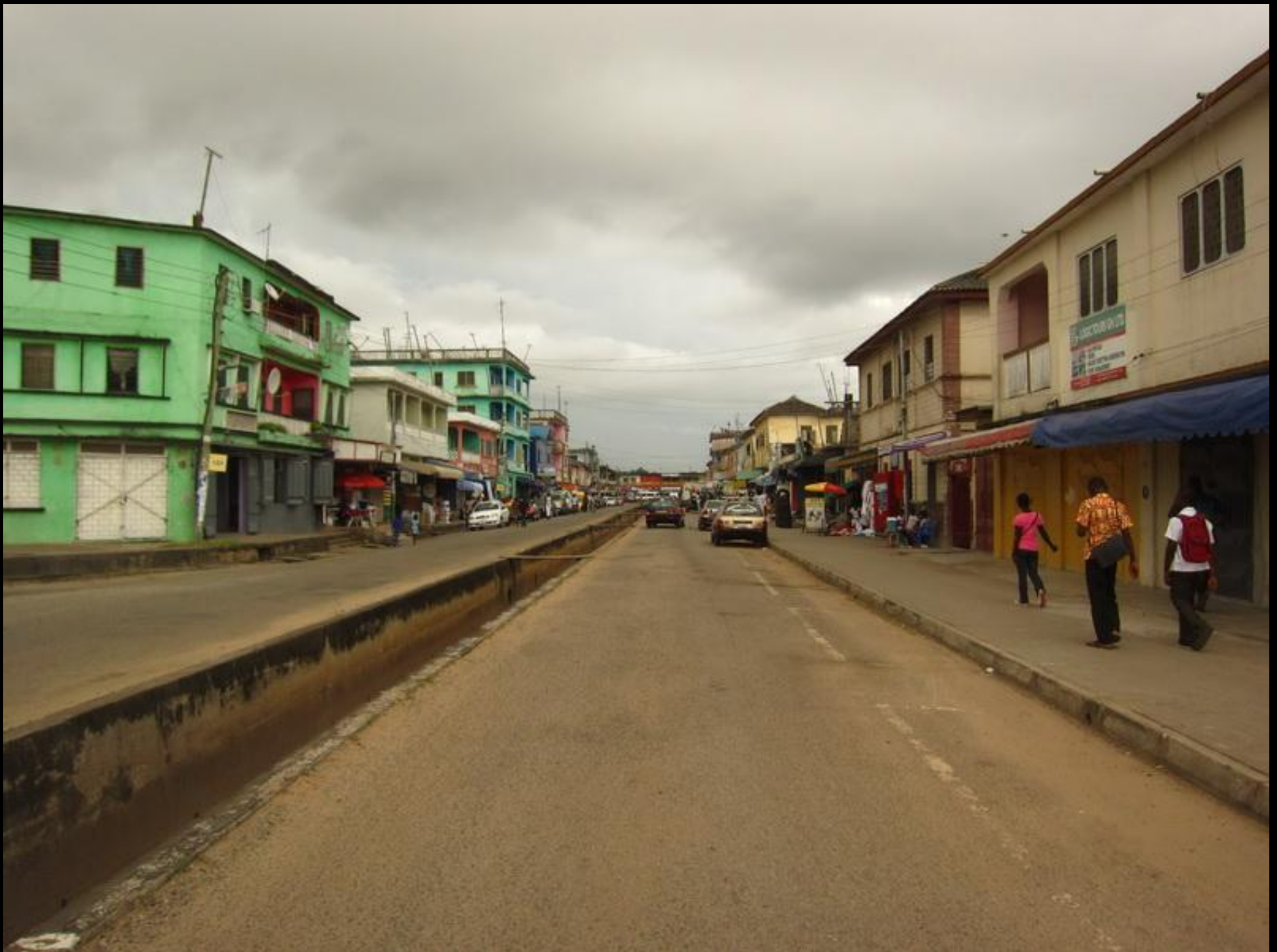
The main street of Takoradi has a large open drain running down the middle of it.
