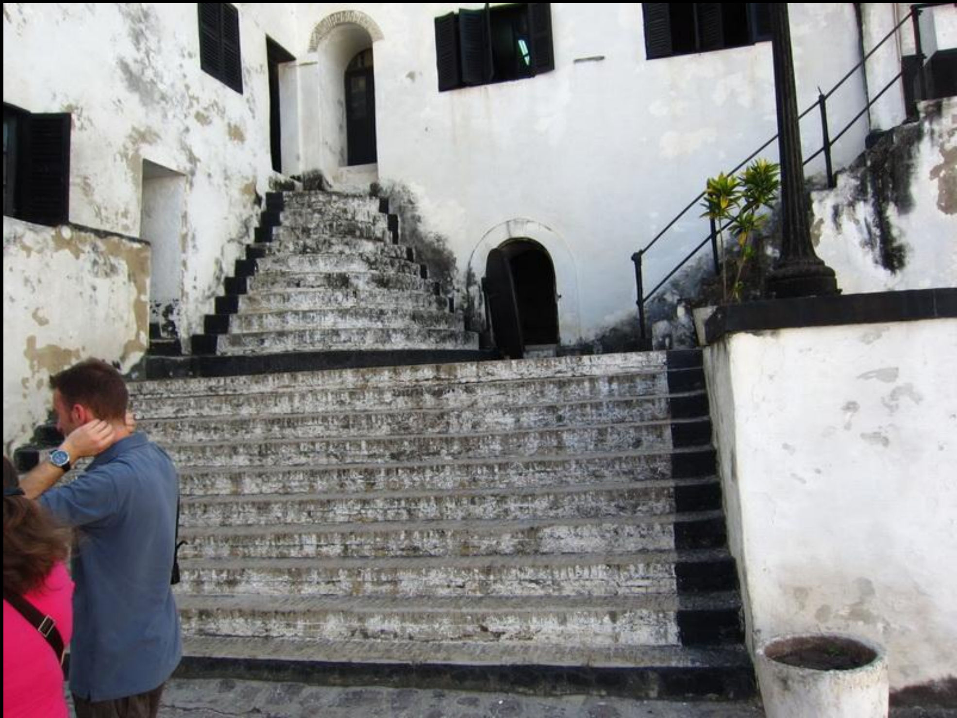
These were the steepest stairs I've ever climbed. No ADA here - no handrails!
