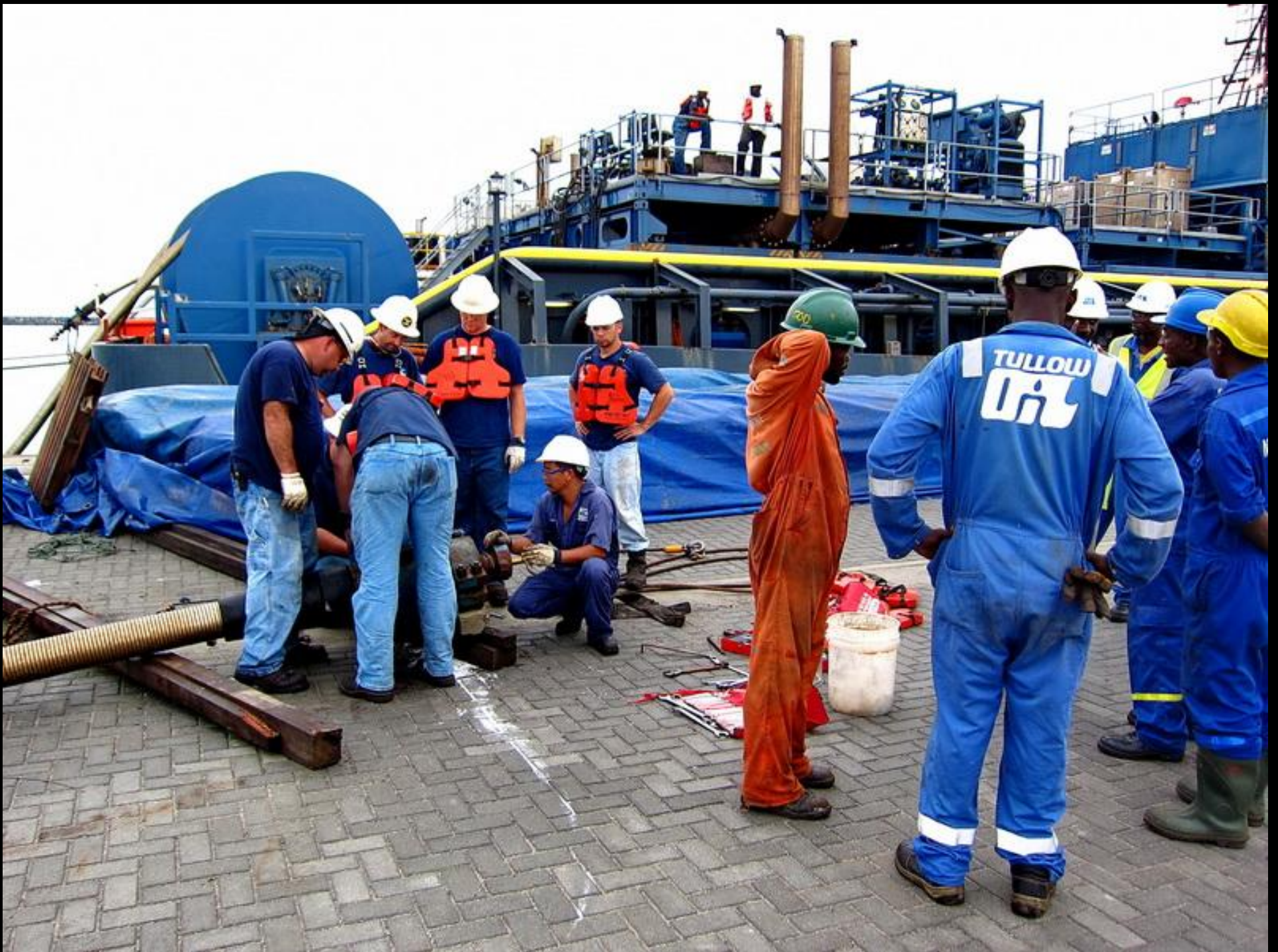
Baker Hughes is overhauling the coflex hanger on the dock.
