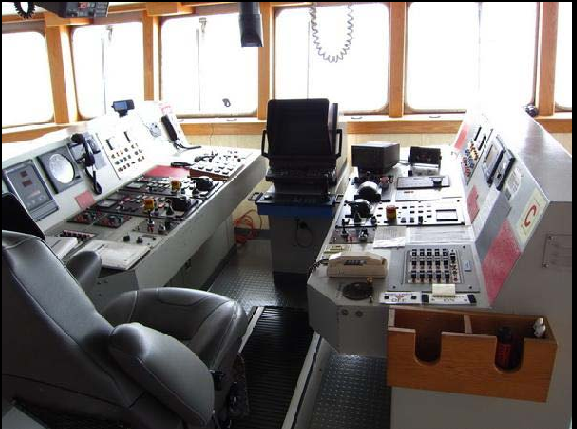
Here are the controls of the forward control station.
