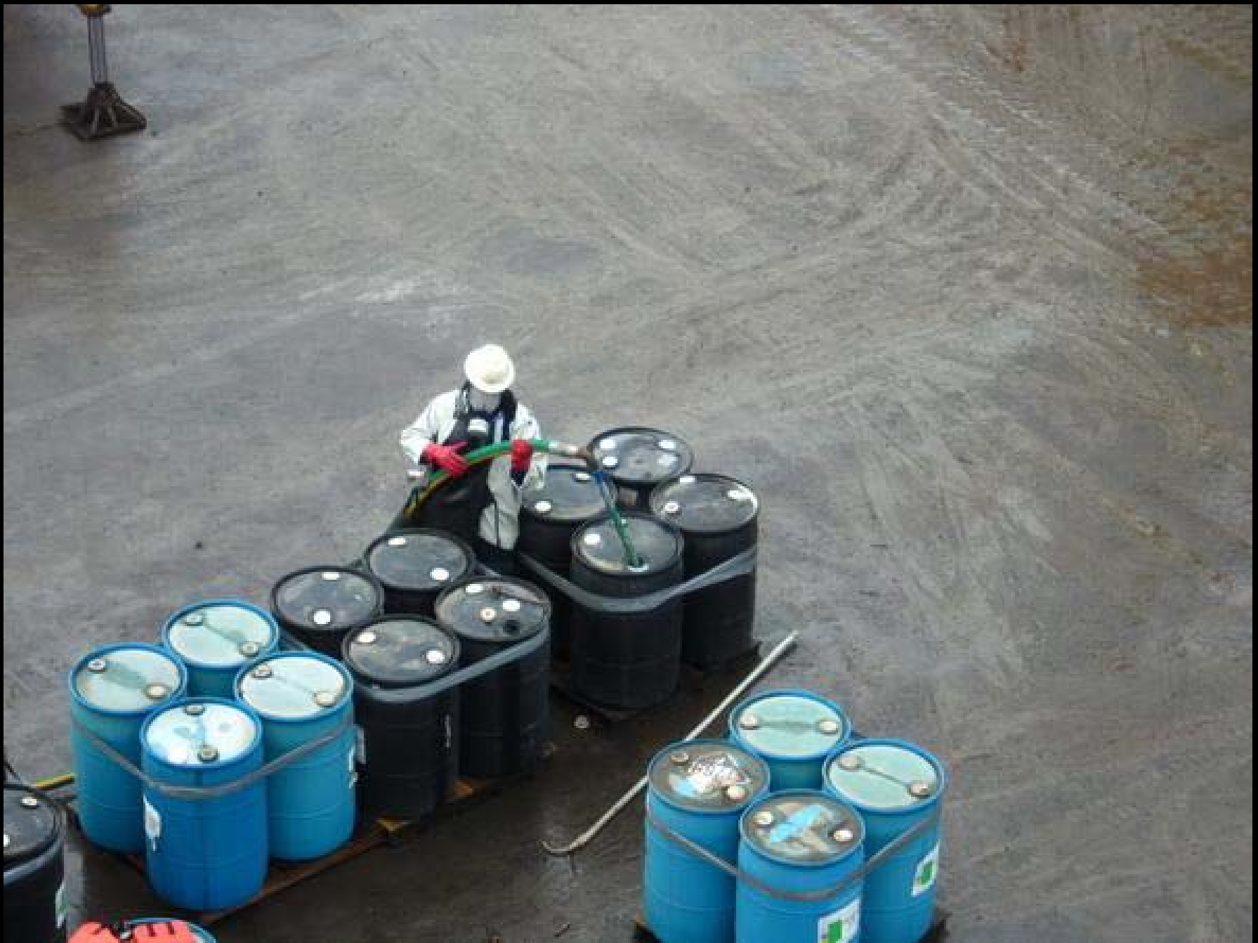
Some of the chemicals used are very dangerous and require some serious PPE (Personal Protective Equipment). This is acid used to pickle the interior of the well bore.
