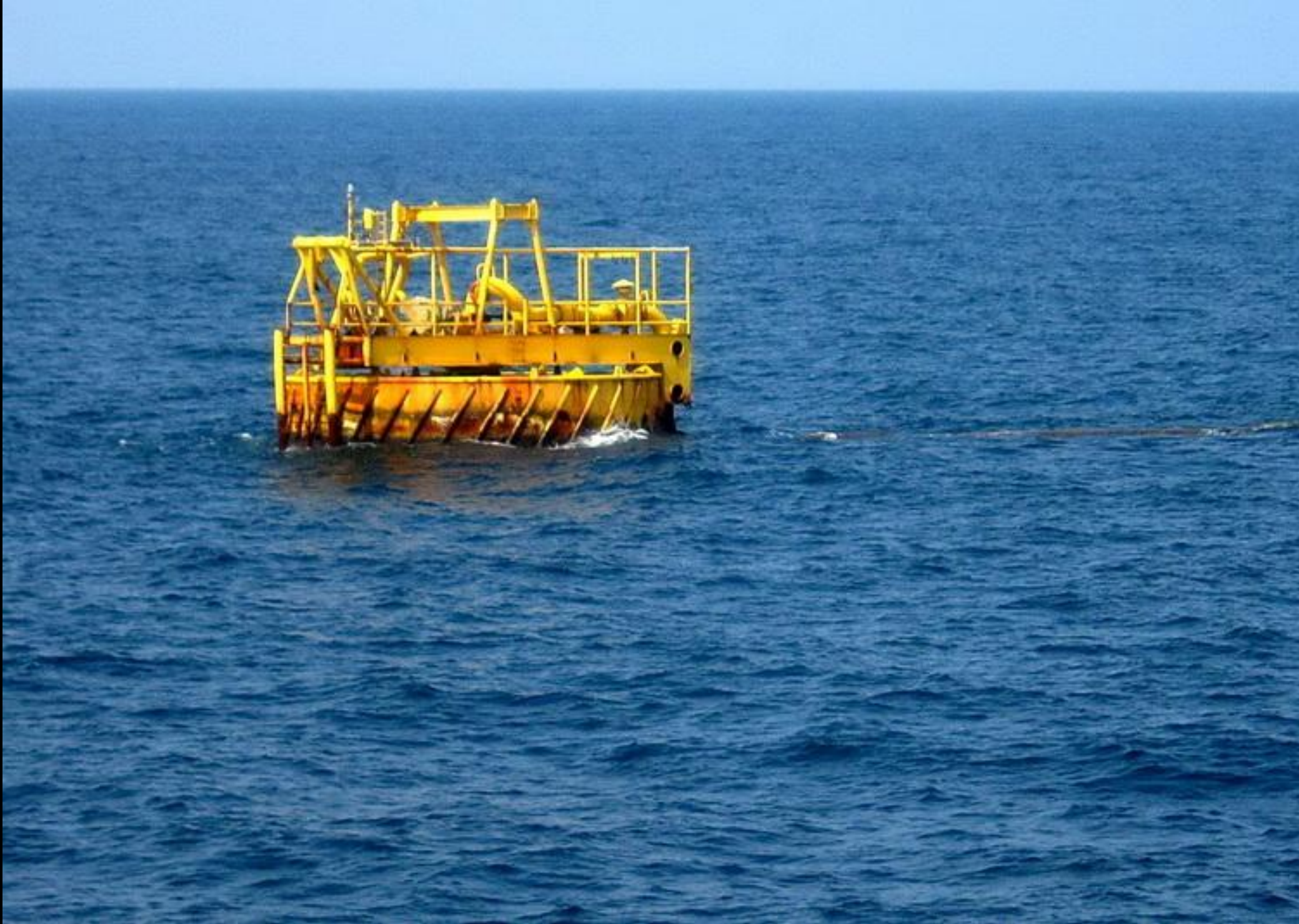
This is the mooring buoy used by the transport tanker. Look at the loading line floating in the water to the right of the buoy.
